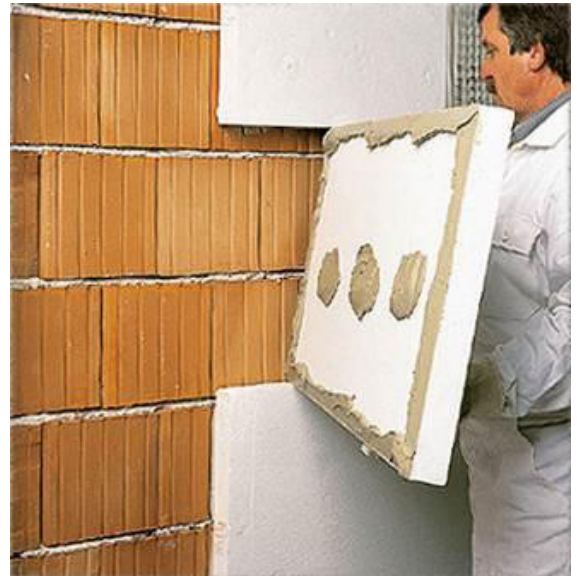
Fig. 1 - Example of Isover EPS 70F application
