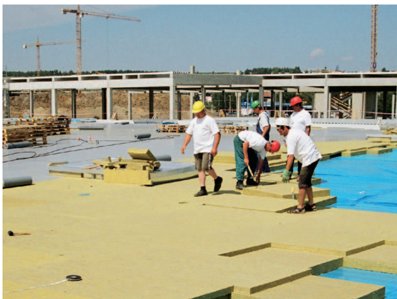
Fig. 1 - ISOVER S as a top layer on flat roof mineral composition.
